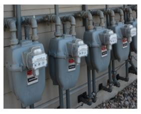
Technology continues to be a component to further enhance processes and customer service. As of August 2018 AMI natural gas modules had been installed on approximately 96% of customer meters. These gas modules communicating through SaskPower's AMI system, and are sending automated meter SaskEnergy's billing reads to Manual meter reads are no longer required for these customers. SaskEnergy meter
