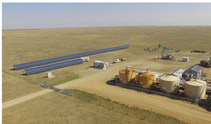
Crescent Point's 100kW solar project
