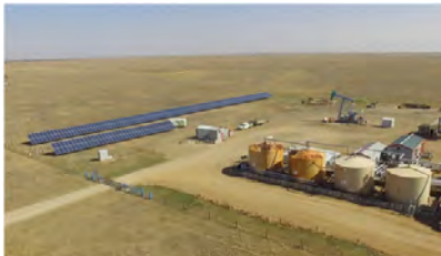
Crescent Point's 100kW solar project
